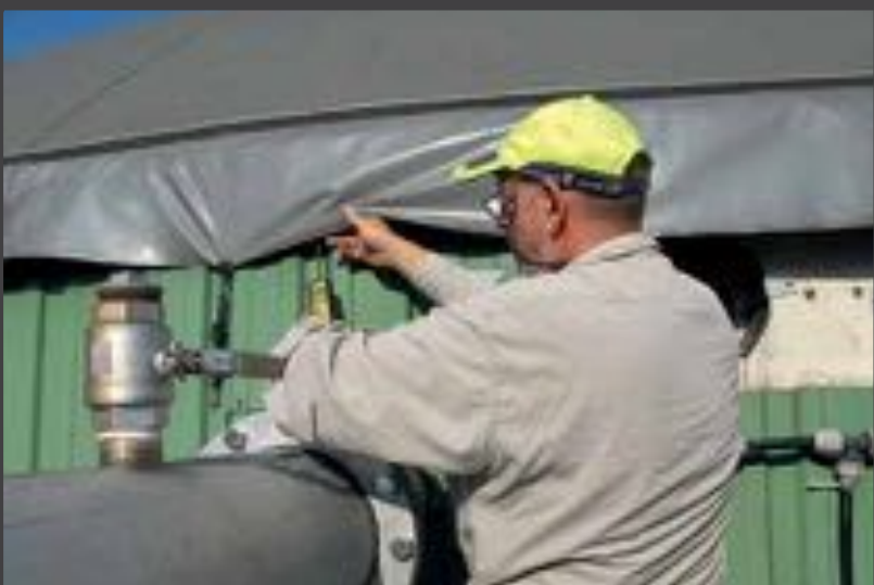
The owner should also check under the edge of the foil regularly. Mechanical wear can be the cause of leaks in the transition area from the digester.
