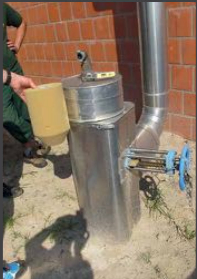
Such a "go-devil" is a tool to clean the pipelines from time to time.
