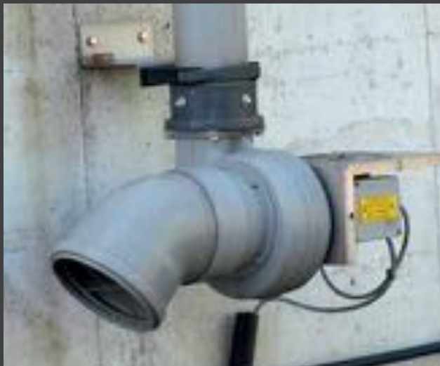
In addition to the portholes as such, all bolted connections should also be inspected.
