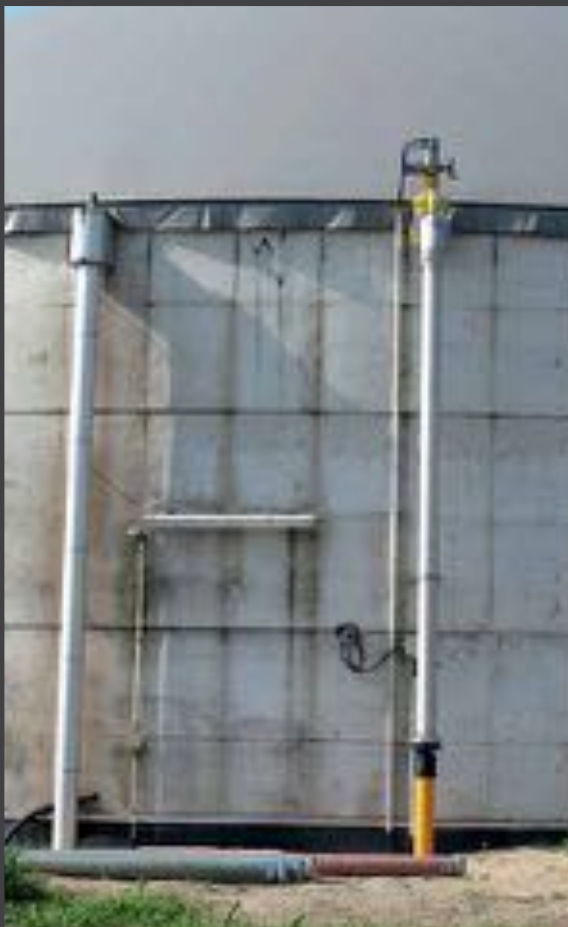
The gas pipeline from the post-digester should also be inspected.
