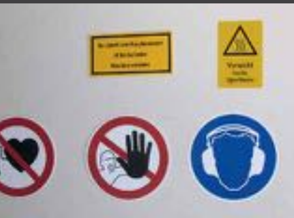
Warnings instruct visitors to wear ear protectors. Especially during open-house days, visitors with a cardiac pacemaker should be told not to enter the cogeneration unit room.
