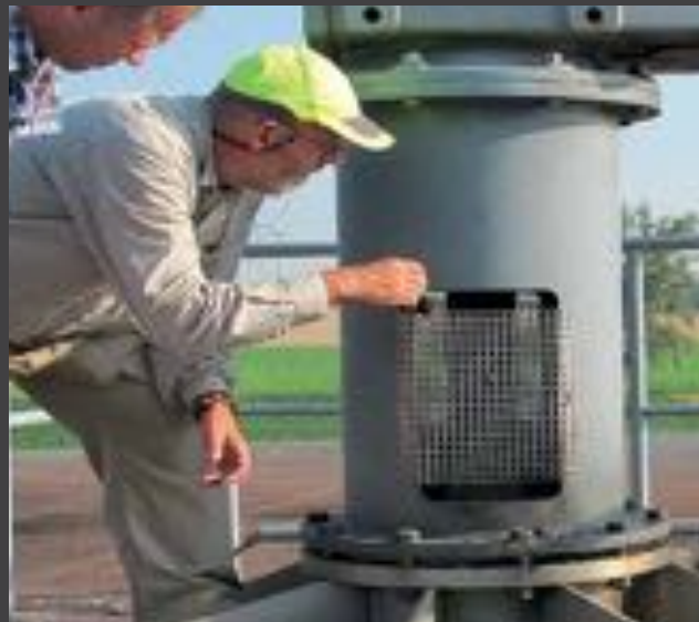
The external parts of an agitator should be inspected closely for dirt build-up and possible corrosion.
