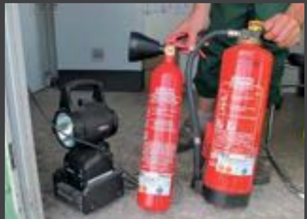
Fire extinguishers (also with CO 2 ) in good working order should be available in every plant, also a lamp for use in potentially explosive atmosphere.
