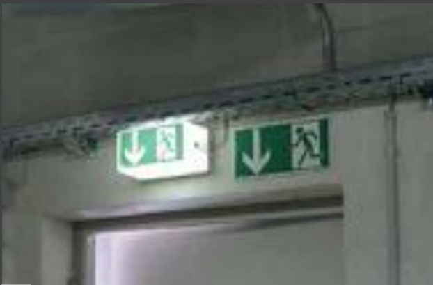
Self-luminous signs marking escape routes are prescribed by law.
